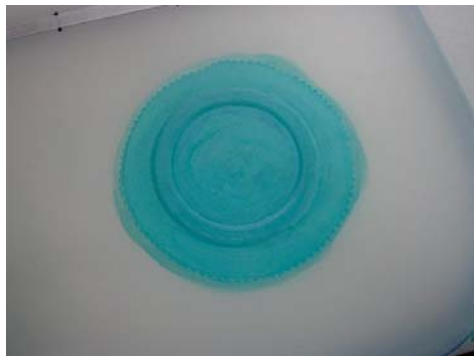
Figure 17-20 - Inspection ring patch glued down.
