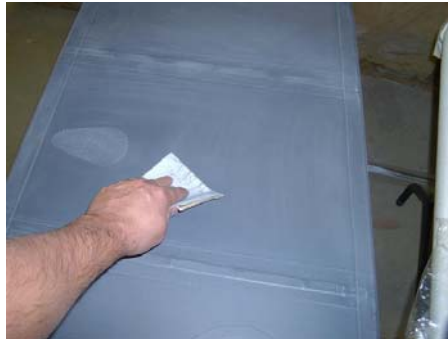
Figure 17-38 - Light sanding with 320 grit open coat paper.
