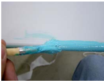
Figure 17-8 - Apply EkoBond for second side, up to the pencil line.
